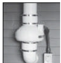
The exhaust fan creates a vacuum to pull radon and other toxic gasses off the water and from the water storage container
